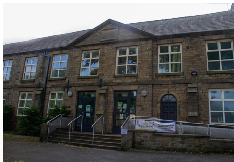
St. Peter's Parish Centre
